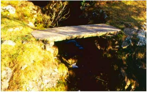
Features of the ancient trackways in Craven described in Pete Shaw's article on pages 30 & 31. Above: The slate slab spanning How Beck on the Stainforth to Helwith Bridge path.
