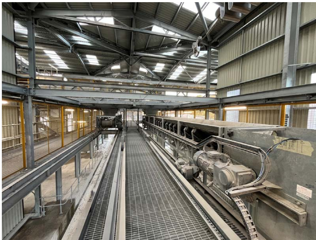
A view inside the new rail loading building.
