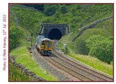
**1.3 Blea Moor Tunnel (north portal):** The wooden platelayers' hut, pre-fabricated concrete fog hut and telegraph poles have been removed and the banner repeater signal has been replaced with a modern colour light signal. Jointed track and wooden sleepers have been replaced by continuous welded rail on concrete sleepers.
