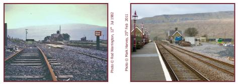
**1.2 Ribblehead station:** The headshunt for the quarry sidings has been moved and a new down platform and waiting shelter have been constructed in its place allowing northbound trains to stop here once more. Replica heritage lighting has been installed on the platforms and the renovated main station building is now a museum / visitor centre. The goods office / weigh-house has been demolished and the goods yard is now a storage area for the Permanent Way Department.
