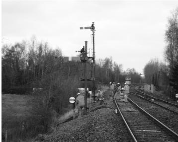
Construction company Eric Wright Civil Engineering installed new semaphore signals at Howe and Co's Sidings during April; they are in the foreground and replace the tall 'bracket' sianal behind. Also visible is Howe and Co's sidings signalbox which was installed by the Midland Railway in 1912 and which is expected to survive for a time after the closure of the rest of the S&C's signalboxes.
