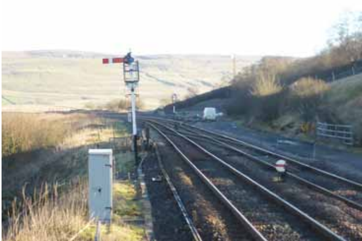
Picture taken from the down platform at Garsdale showing the crossover, the main line curving to the left and a conveniently parked white van marking the point where the former branch line curves to the right to begin its descent to Hawes.
