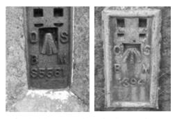
Left: Flush bracket at 'Vicar's Allotment'. Right: Flush bracket at New Bridge.
