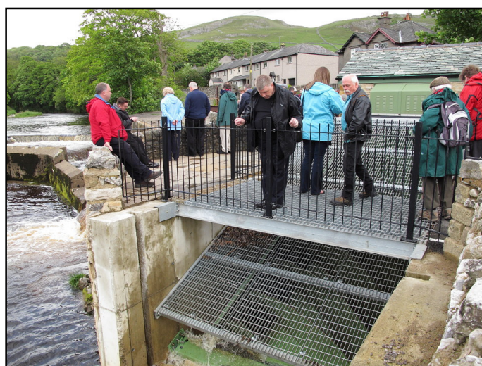
16: The Settle hydro-electric generating plant
